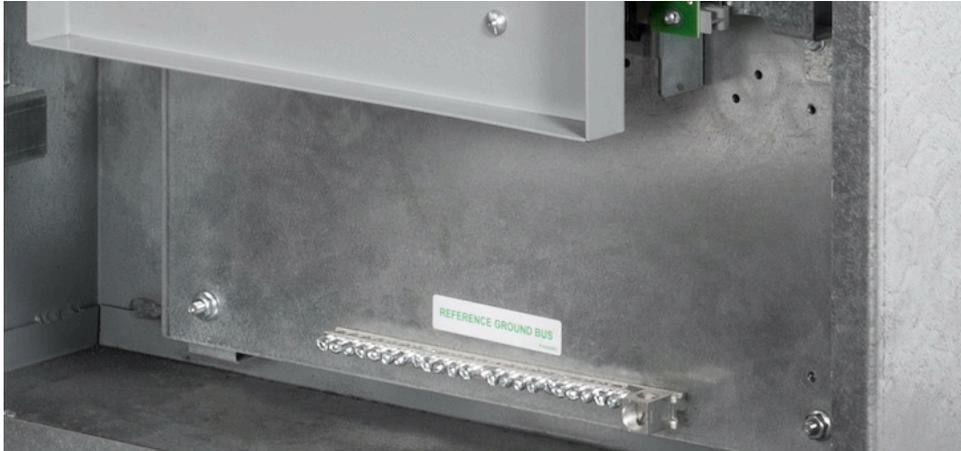
Connect all ground conductors from the equipment and receptacles in the area served by the isolated power system to the panel's ground bus.
