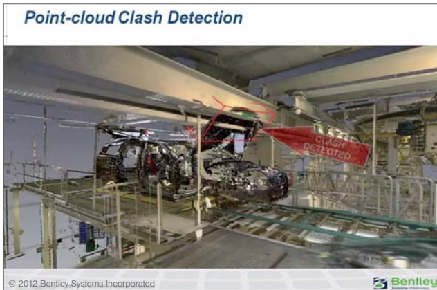
Data from product development and scanned production site is used for collision checking.
